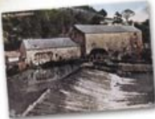
Bridge End Mill
