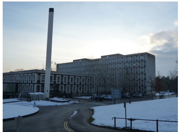
Existing Flintshire County Hall buildings
