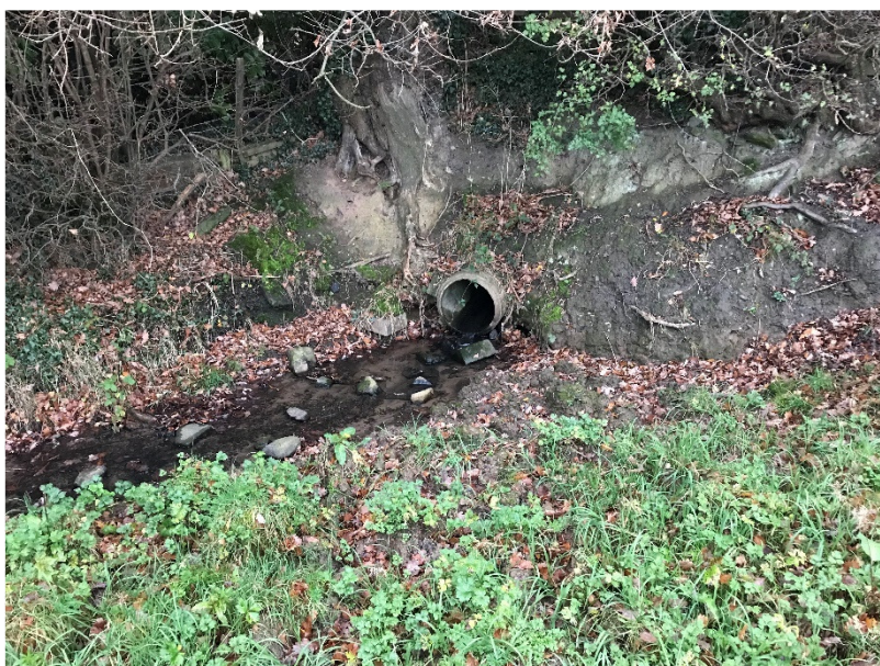
Figure 3: image facing to the south (upstream) of the watercourse as it emerges from a culvert passing beneath a finger of land extending into the site along the eastern boundary.
