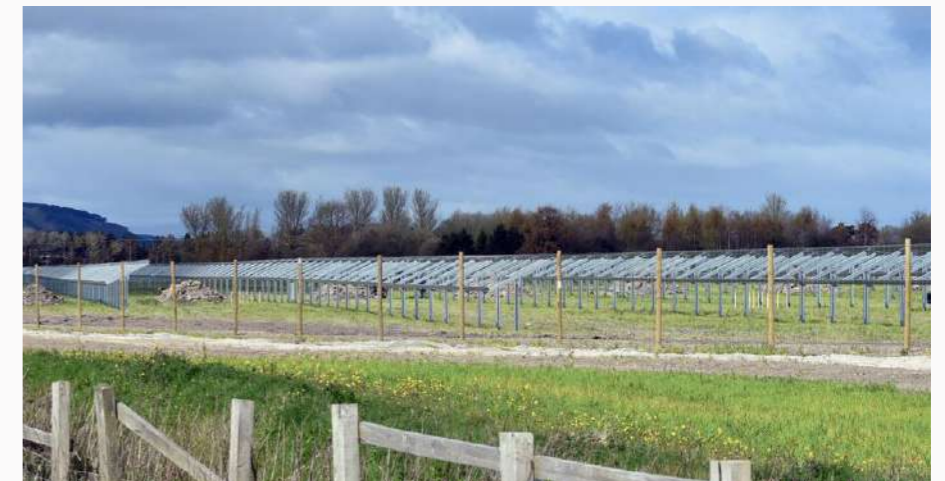
Figure 4. Typical view of solar farm during installation
