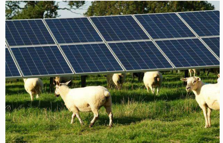
Figure 3. Appearance of solar panels
