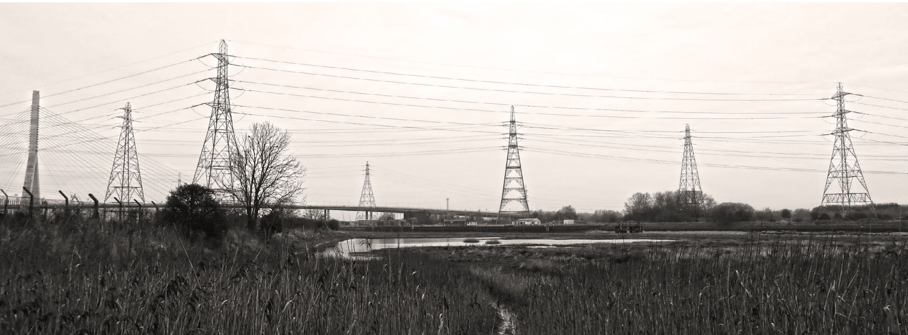
Fig 5.01: View of the site
