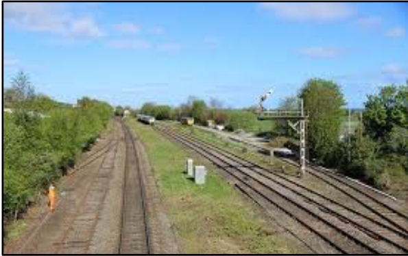
View towards Mostyn, from Dock Road Bridge. The two running lines next to the wide green strip (former platform) will be kept and all other
