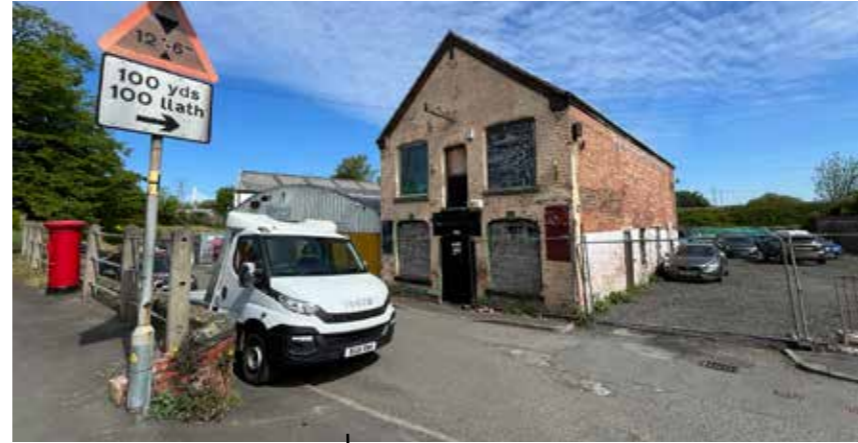
Vacant/derelict building creating an unattractive gateway.
