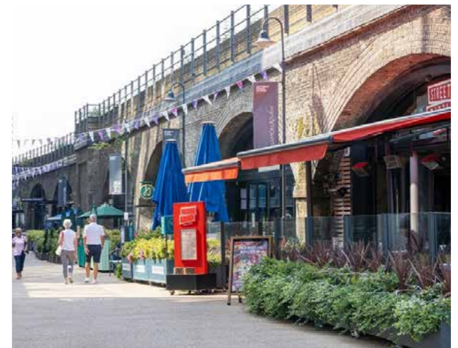
Make the most of existing assets
