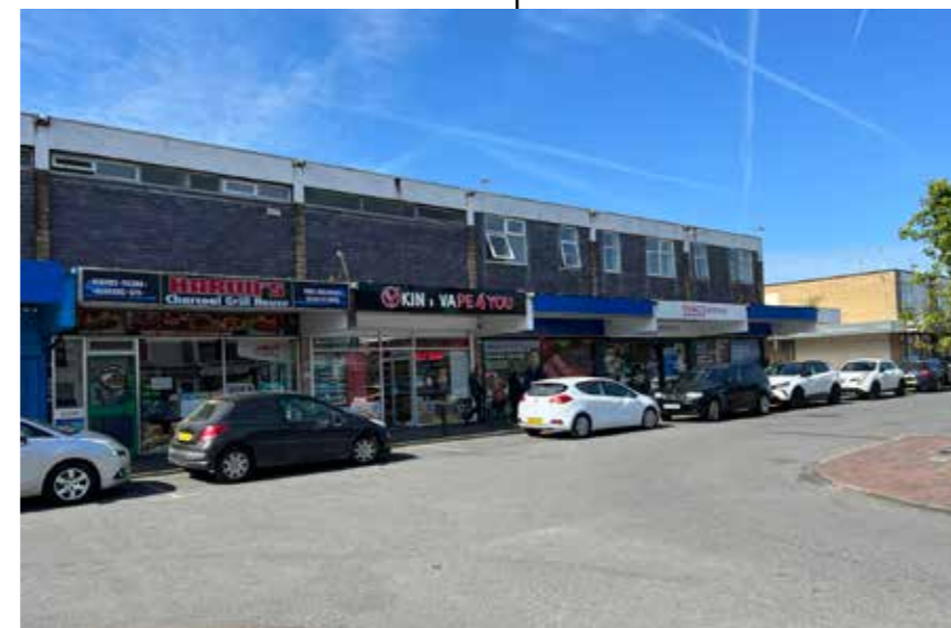
The Precinct consists of a large amount of space used for car parking creating a vehicle dominated environment in a prominent central location.
