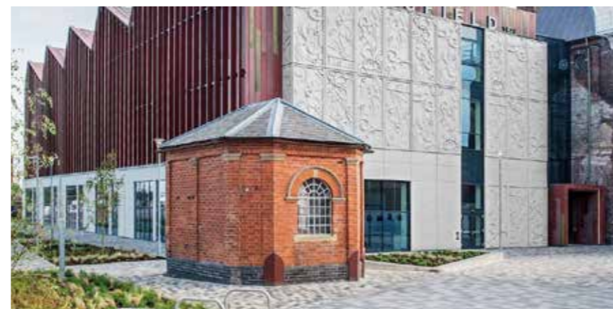
Reuse derelict buildings
