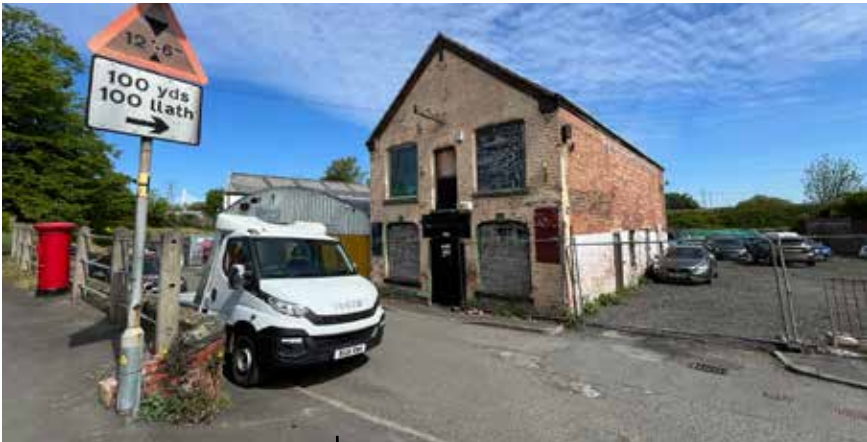
Vacant/derelict building creating an unattractive gateway.
