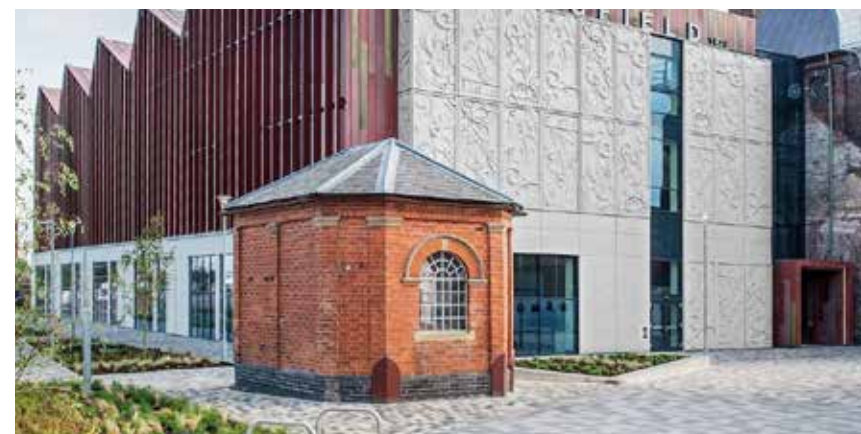
Reuse derelict buildings
