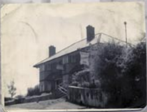
The new Crown Inn
