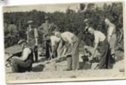
Volunteers digging the foundations for Pantymwyn Village Hall
