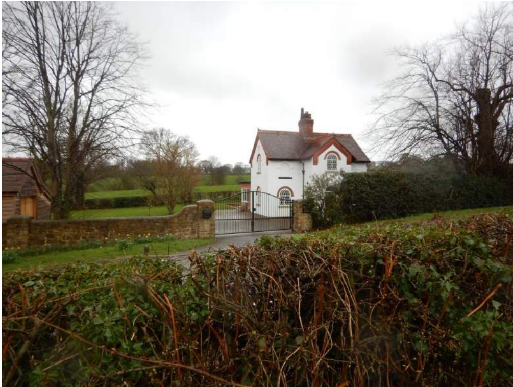
Photograph 15: View of Hillside Cottage at southern edge of site.
