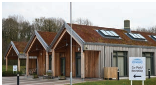
ENGIE headquarters, Mold
