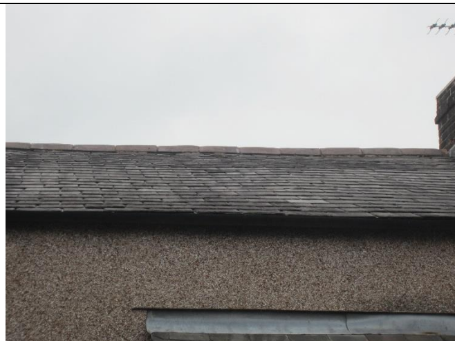
Photo 14: Gaps for bat access beneath the ridge copings at Ivy Cottage
