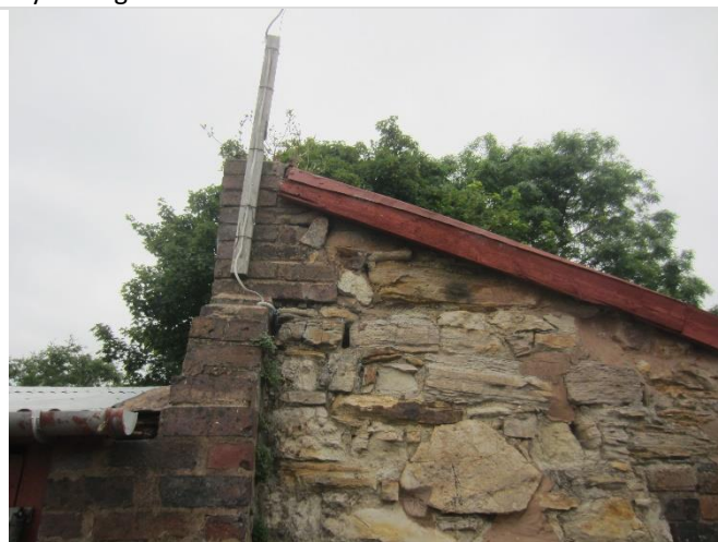
Photo 16: Gaps in the stone elevation wall at Building 2
