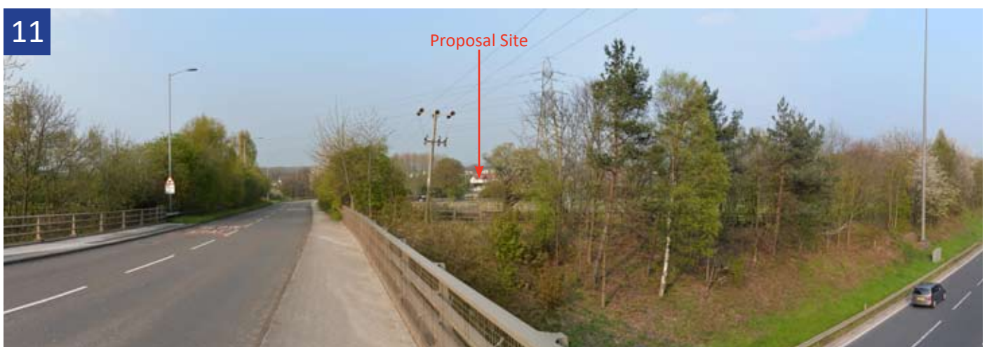
Photo from Liverpool Road at bridge over the A55. Views north are partially screened by trees along the roadside of the A55. Glimpses of properties Liverpool Road and Mold Road are possible with fields beyond.
