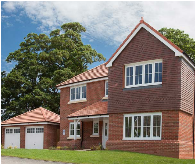
Photograph taken from the Anwyl Homes development Parc St Marys, Northop Hall
