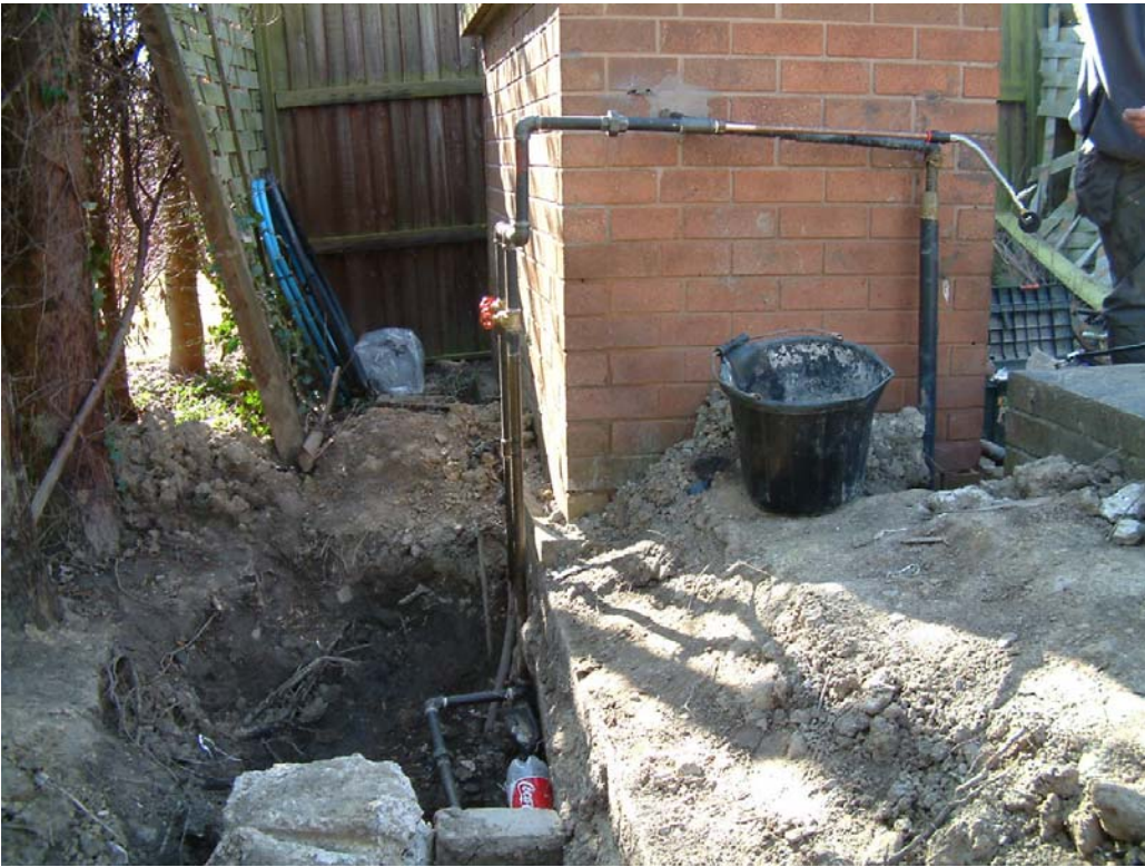
PHOTOGRAPH 4 NEW SUPPLY PIPE WITH PRESSURE METER ATTACHED
